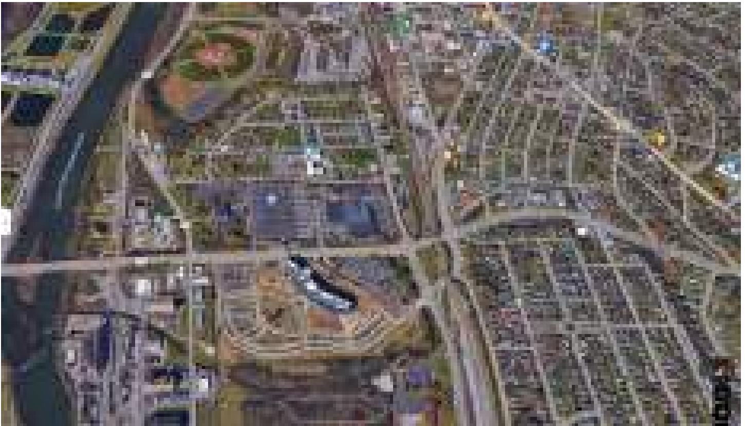
Eastman chemical recycling facility in Kingsport, Tennessee. Source: Google Maps
